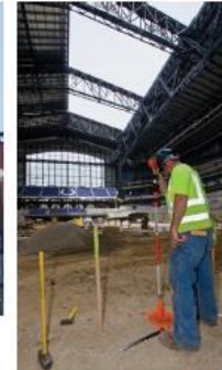
Control points were set in front of the base of the steel SuperFrames on the north end of the stadium and corresponding control points were set at the other end of the stadium, as well as just south of the 50-yard line in the middle of the playing field.
